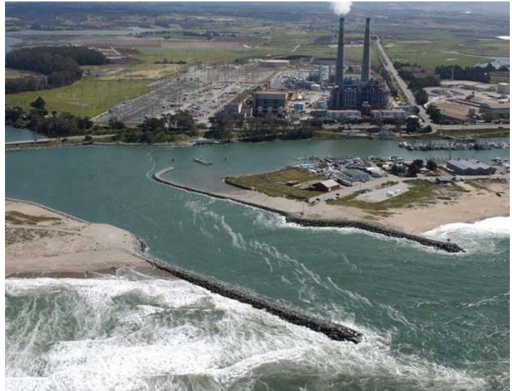
Figure 2. Moss Landing Harbor levees
