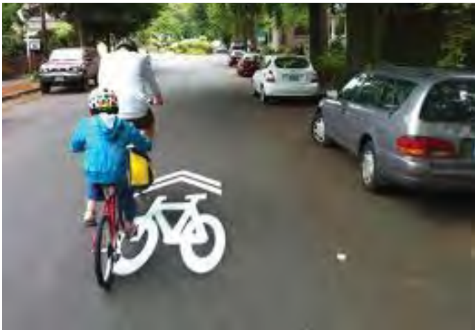
A narrow roadway with sharrow markings encourages slower speeds and is more comfortable for bicyclists.
