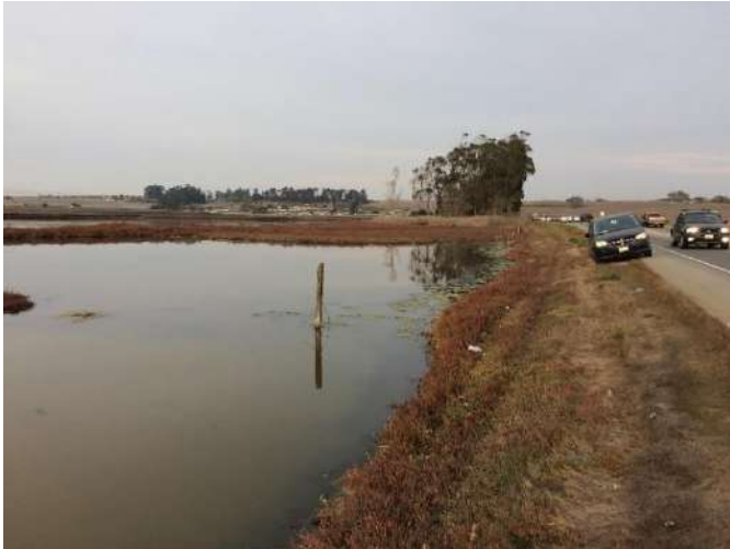
Reach 1 culvert located underneath vegetation)
