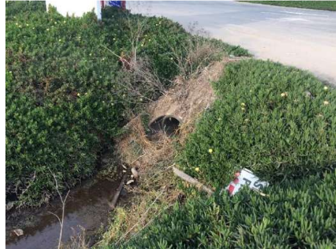
Reach 2 culvert by Bennett Slough
