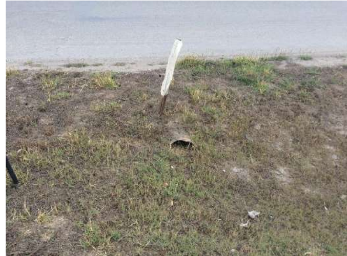
Reach 4 culvert (note structure is filled in)
