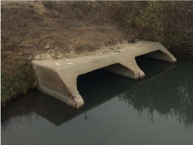
Reach 3 dual concrete culverts
