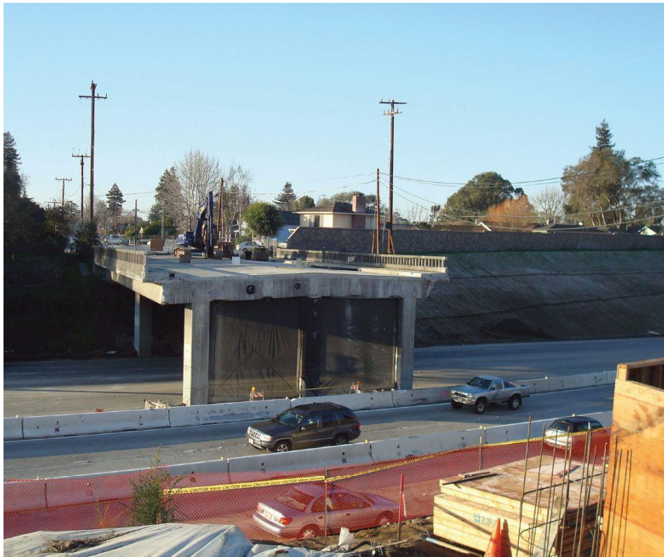
Road Construction, Santa Cruz County
